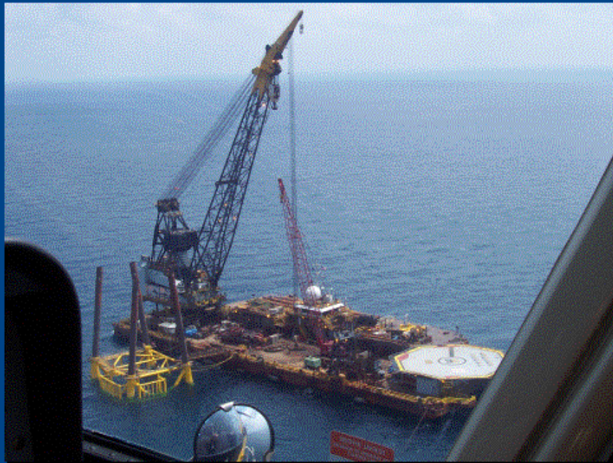
Horizon Derrick Barge "Pacific" setting A5 Jacket
