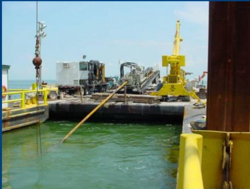
24" Pipeline Horizontal Directional Drill Site on Galveston Bay Water to Water drill under the Texas City Dike & Ship Channel
