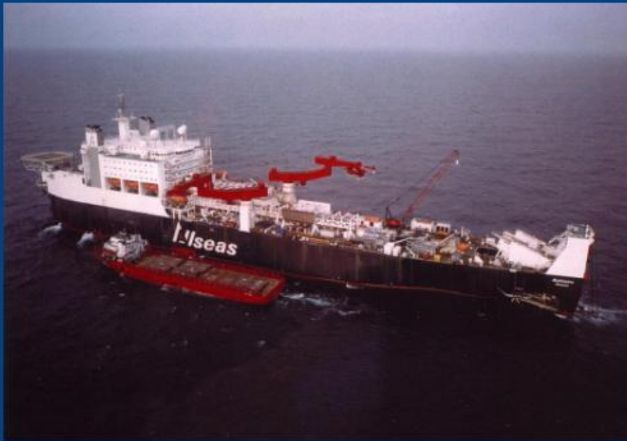
Pipelay vessel 'Solitaire' in the process of laying the 30-inch pipeline
